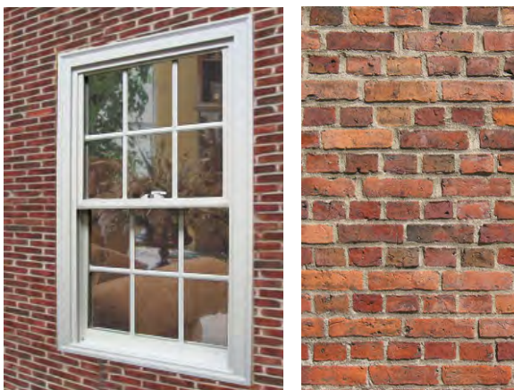
EXISTING BRICKED WALL TO BE CLEANED, REPAIRED AND RE-POINTED. ALL WINDOWS TO BE REPLACED.
