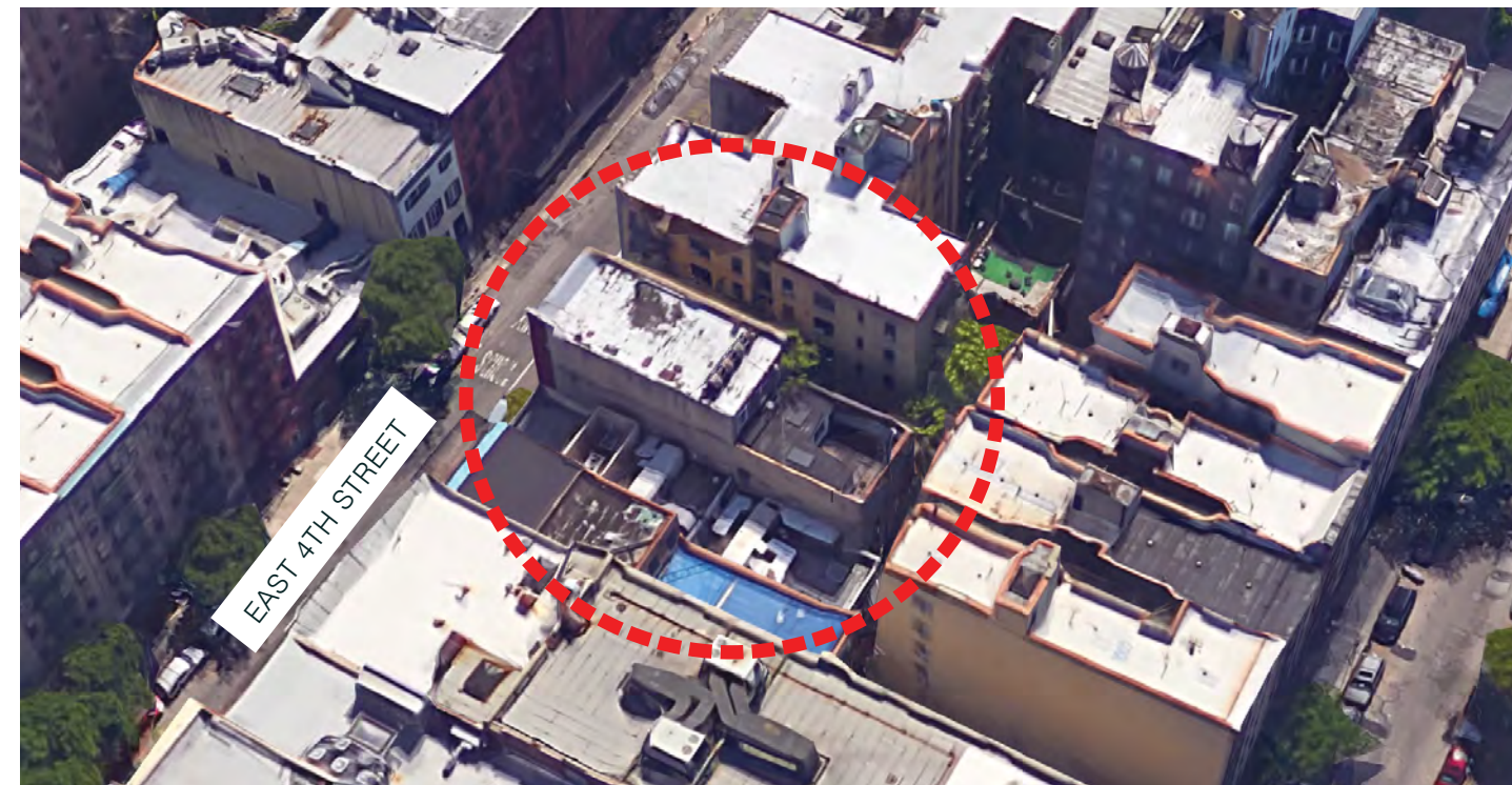
AERIAL VIEW FROM SOUTHWEST
